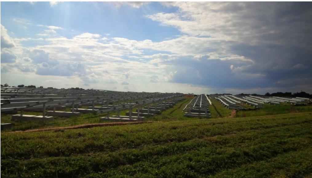
Photo 14: Racking System installation, Parklands Landfill, NJ. Note concrete ballast
